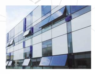
**VECOSTA** provides excellent acoustic performance (between RW 45 and RW 49). A real asset for technically advanced and design-focused facades.
